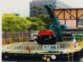
取水人孔（施工例）①
